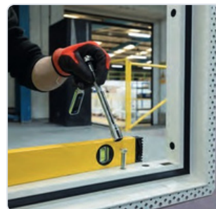
PRECISION adjustable frame aligned on site — no packers, no mastic
